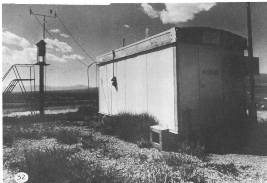
Figure 32. Perimeter monitoring station at CAMDS
